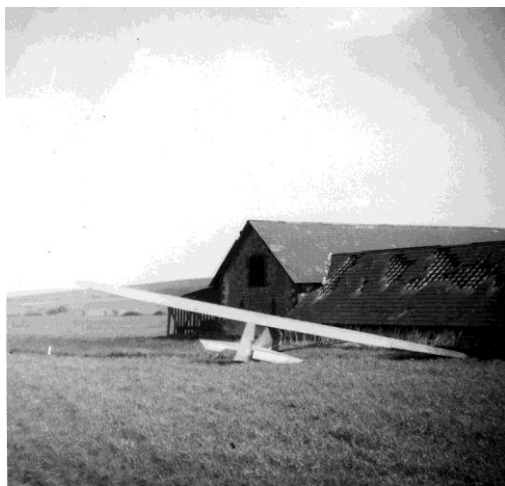
Outbuildings from south west
